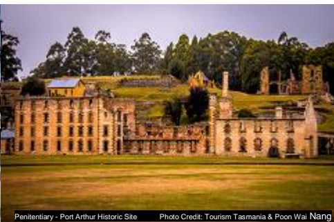
Penitentiary - Port Arthur Historic Site
